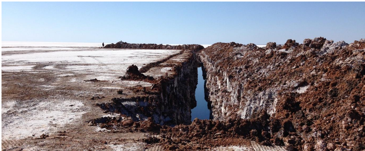
Figure 3. Trench at MT1
