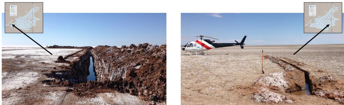
Figure 1. Trenches and Field Tests Completed
