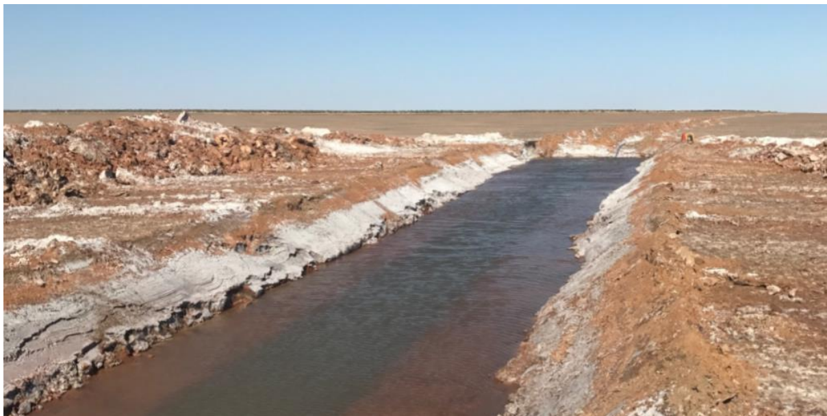
Figure 1. Trench T9 Prior to Commencement of Pump Testing
