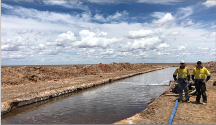
Shallow Water Table for Trench Brine Extraction
