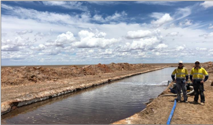
Shallow Water Table for Trench Brine Extraction
